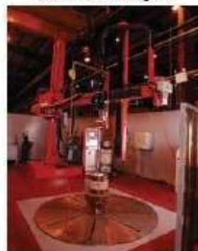
HotWire Tig Cladding Installation for overlaying of internal and external valves.
